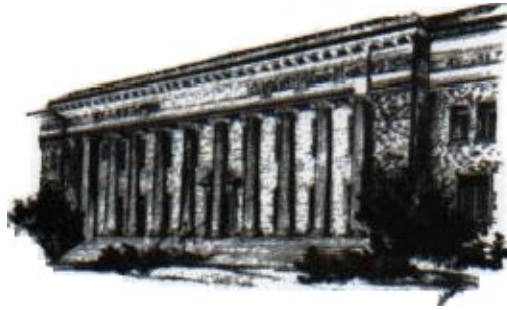
Tehama County Courthouse
