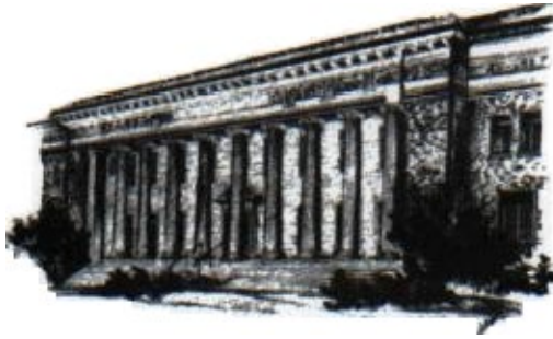
Tehama County Courthouse
