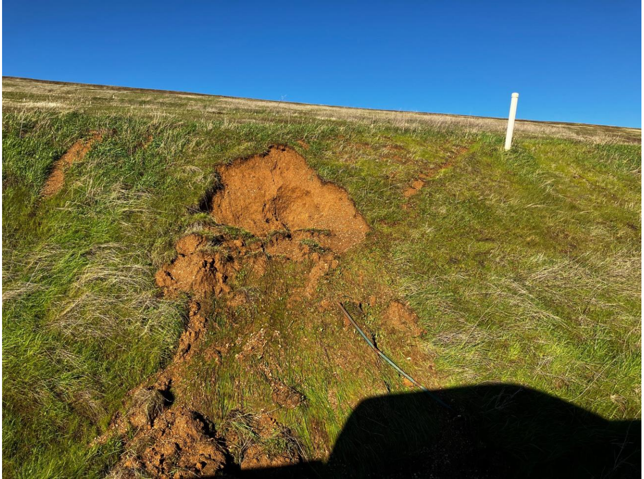
Figure 3: Phase I Southeast Slope erosion (Feb. 2025)
