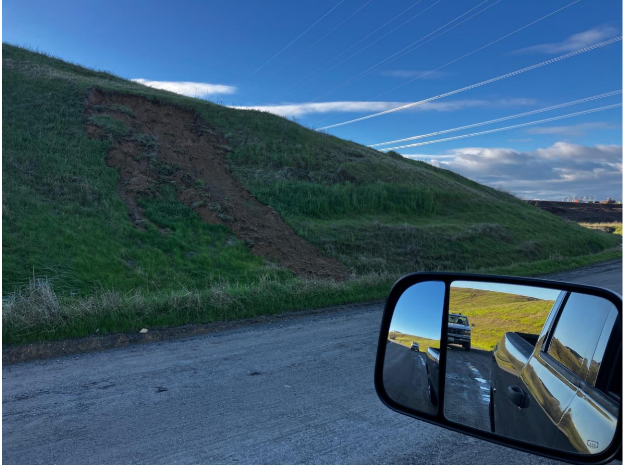
Figure 5: Phase I Northwest Slope erosion (Feb. 2025)
