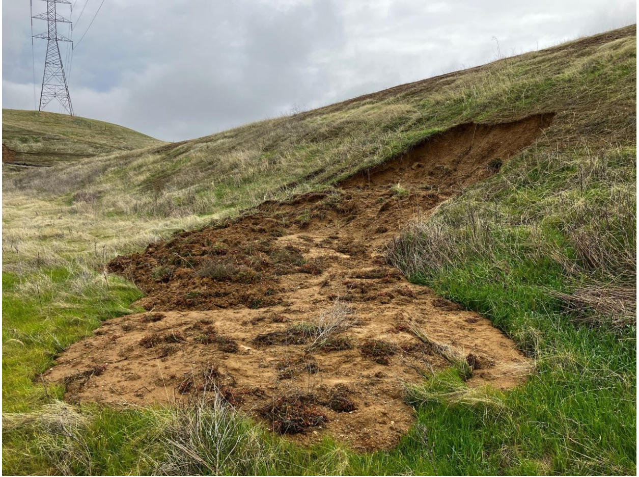
Figure 1: Phase I West Slope erosion (Dec. 2024)
