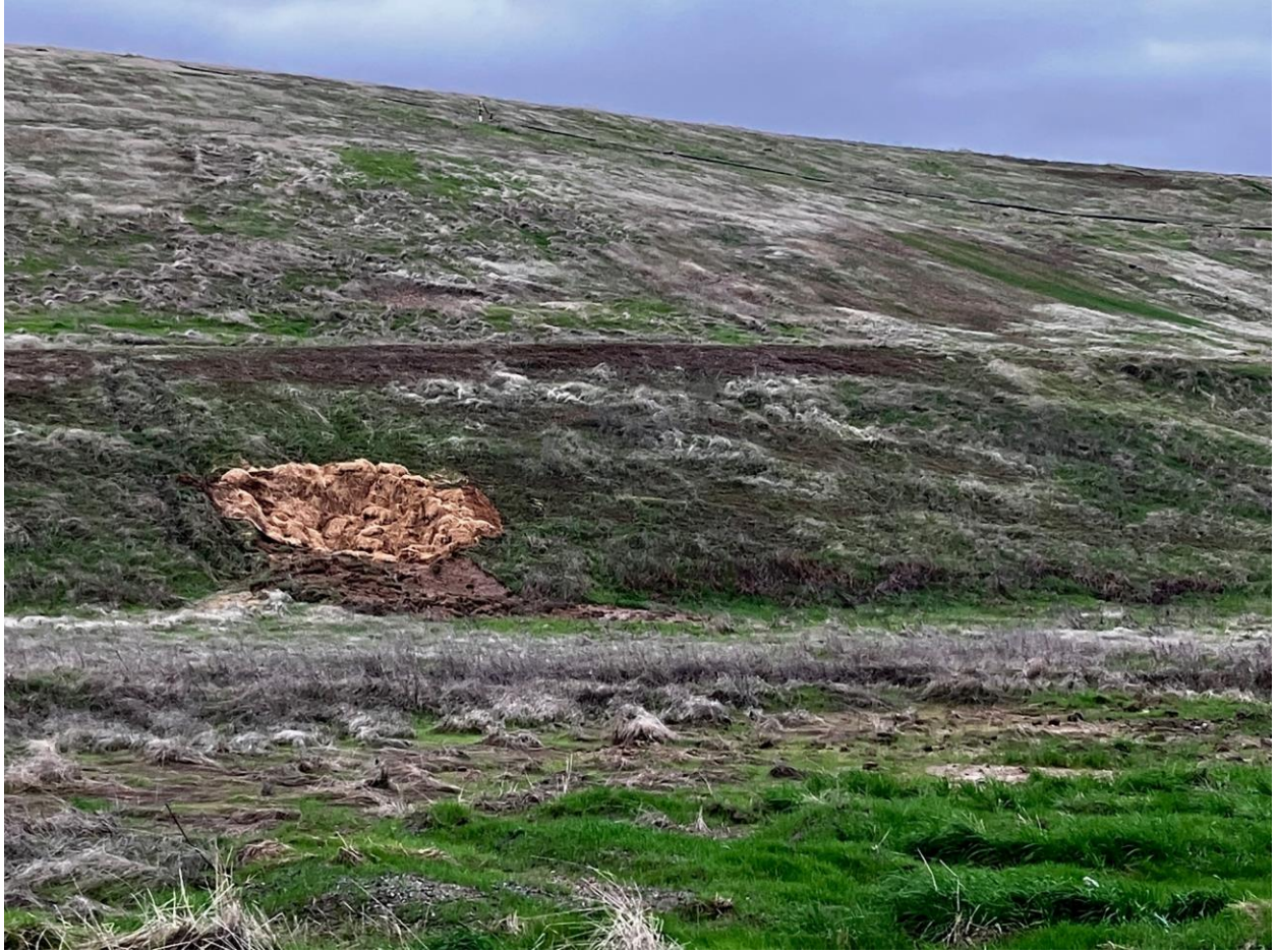
Figure 2: Phase 1 West Slope erosion w/ straw (Dec. 2024)
