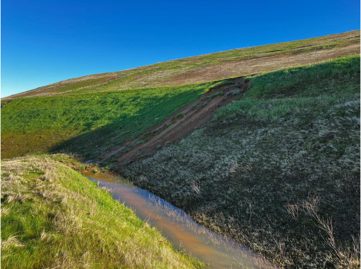
Figure 4: Phase I West Slope erosion (Feb. 2025)
