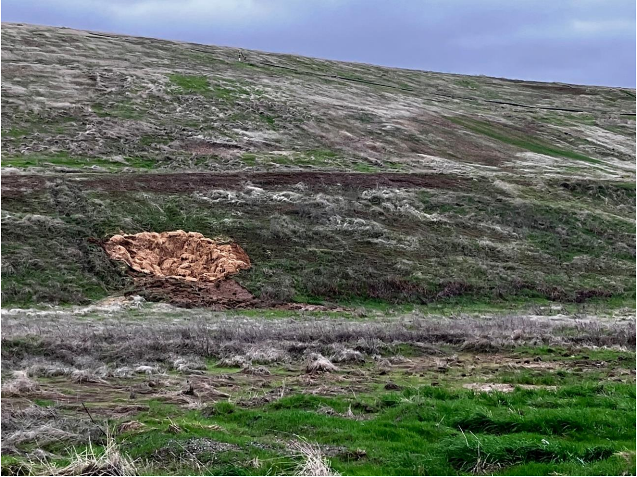
Figure 2: Phase 1 West Slope erosion w/ straw (Dec. 2024)
