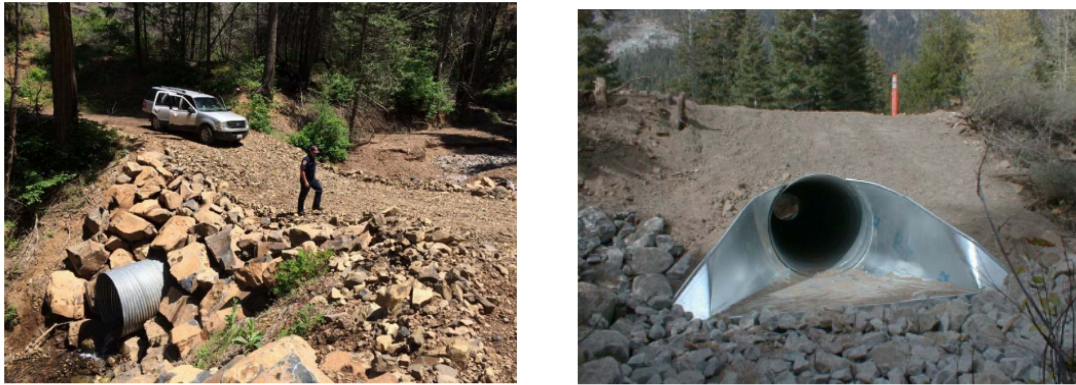
Figure 2: Examples of culvert design interventions to manage debris flow (Source: Cafferata et al., 2017. Designing Watercourse Crossings for Passage of 100-Year Flood Flows, Wood, and Sediment (Updated 2017) )
