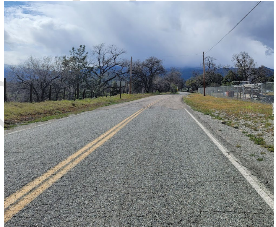
Figure 5 - Current Pavement Condition, Paskenta, CA
